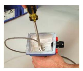
3. Tighten with Screwdriver, Cut Wire to Length
